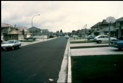
The Drive, Pave and Pipe Approach...
